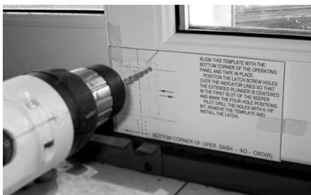
**4** Pilot drill the holes with a 3/32" bit. (Photo #28)
