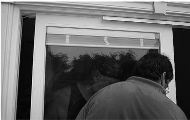
1 Lift the fixed panel up & into the head pocket (Photo #7), swing the bottom in, and set it down onto the fixed panel shim.
