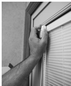
1 Position the external magnet after carefully cleaning the glass area where it will be placed. For proper operation, the external magnet must be perfectly interfaced with the internal one. Therefore, before removing the adhesive protecting film, position the external magnet on the glass next to the internal one. Verify smooth raising and lowering of the blind. Then remove the film and position the external magnet on the glass following the magnetic attraction. (Photo #21)
