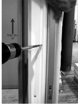
6 Fasten the exterior astragal post to the fixed panel using the 5 - 2 1/2" installation screws in the 5 pre-drilled holes. (Photo 9A)
