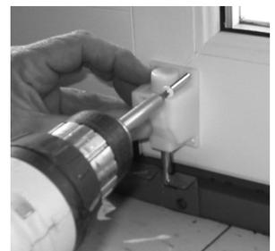
**5** Remove the template and install the latch. (Photo #29)
