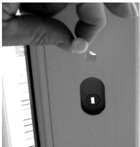
1 If provided, insert grommet into the two interior holes for assembly screws. (Photo #16) Follow the installation instructions in the handle set box using step 1 first, then step 2 for the trim set with the key cylinder.
