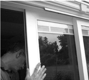
1 From the inside, lift the operating panel up & into the head pocket - swing the bottom in - set it down onto the stainless steel roller track. (Photo #12)
