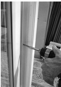
3 Drill three 3/32" holes into the sash using the pre-drilled holes through the frame's center leg. This will help keep the sash from drifting when screwing into place. Secure the fixed panel to the mainframe using 3 - #8 x 1 1/4" security screws. (Photo 5A)
