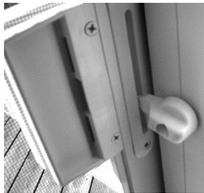
1 Slide the patio door screen closed and, while holding the door closed, rotate the knob into the latch in the face of the screen. (Photo #20)
