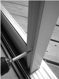
3 Screw the interlock to the fixed panel. Use the 5 #6 x 3/4" flat-head screws. (Photo #9)
