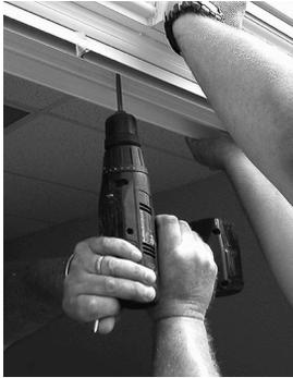
3 It is recommended that 1-2 screws be run into the head through the outer channel of the frame into the home. (Photo #4) Photo #5
