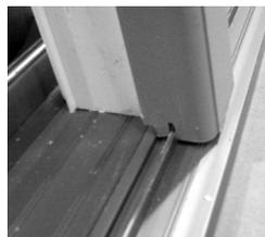
4 Insert the exterior astragal post, positioning the head end first, and taking care to line up the notches on the sill end with the sill track. (Photos 6A & 7A)
