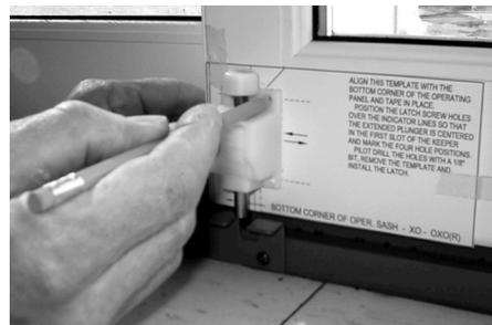
**3** Position the latch screw holes over the indicator lines so that the extended plunger is centered in the first slot of the keeper and mark the four hole positions. (Photos #26 & #27)
