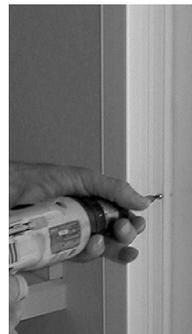
**CAUTION!** Do not install screws to fixed panel (next, step 6) until the operating panel is installed and locked!
