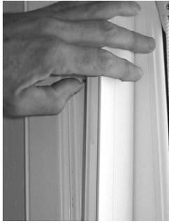
1 Snap in the first pocket cover in the interior channel of the jamb in front of the fixed panel. This covers installation screws as well as the screws that secure the fixed panel in place. (Photo #18)
