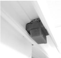
4 With door closed, mark head rail (with pencil) at meeting rail edge for T-Foam placement. Remove door and attach T-Foam, adhesive side up, to head rail at marking (Photo #13A). Reinstall operating panel.
