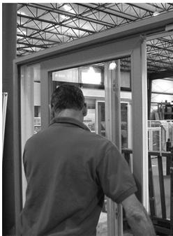
1 Lift the fixed panel up & into the head pocket (Photo 3A), swing the bottom in, and set it down onto the fixed panel shim.
