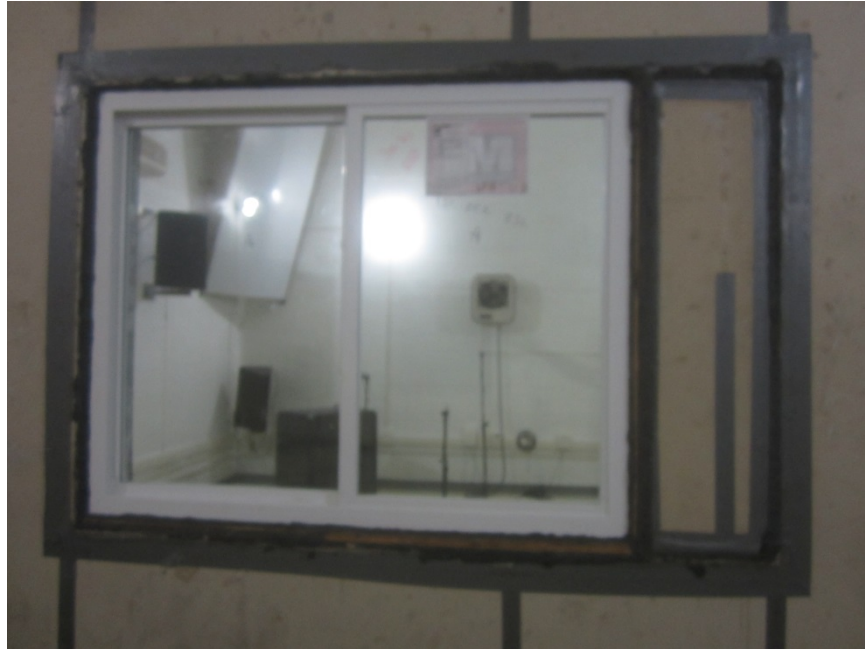
Receive Room View of Installed Specimen
