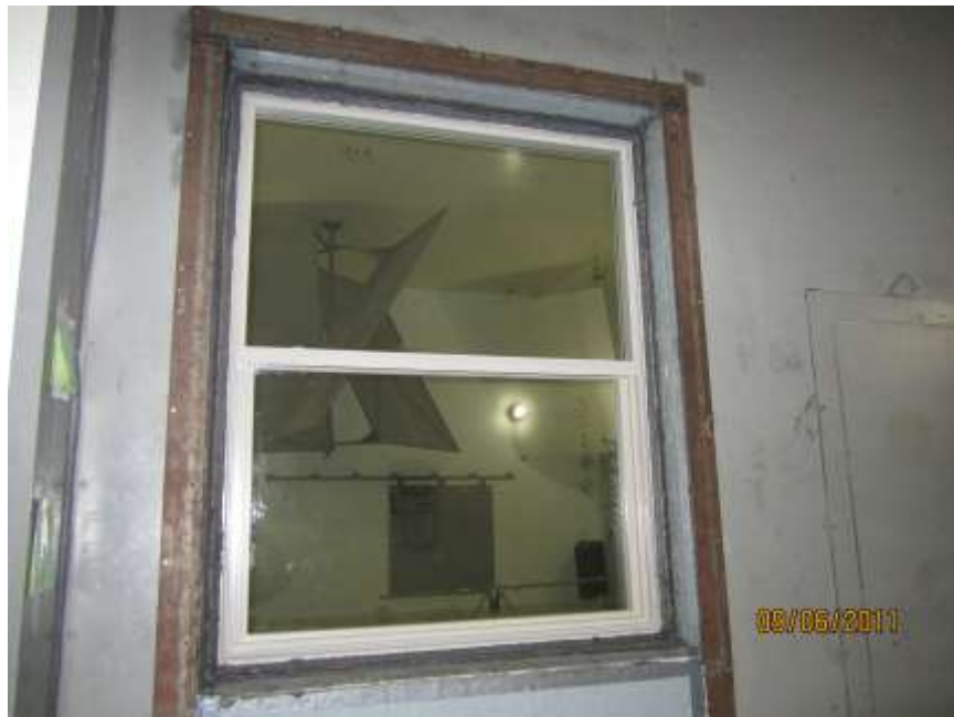
Source Room View of Installed Test Specimen
