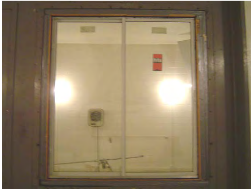
Receive Room View of Installed Specimen
