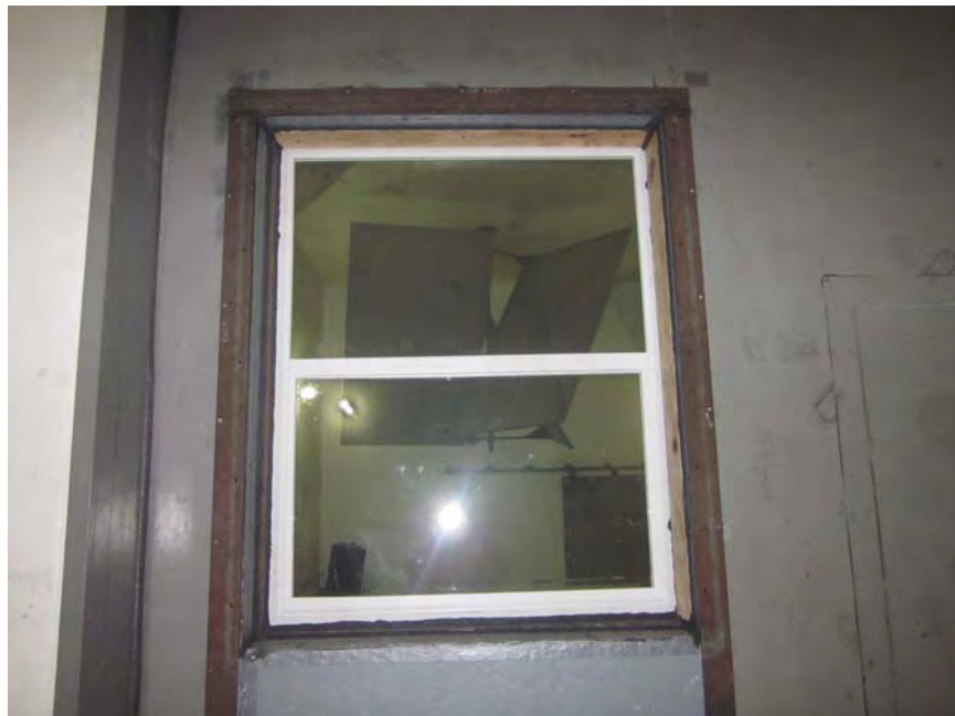
Source Room View of Installed Specimen
