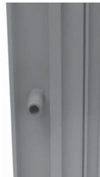
Astragal with bumper installed
