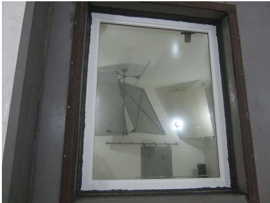
Source Room View of Installed Specimen
