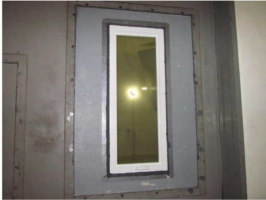
Receive Room View of Installed Specimen
